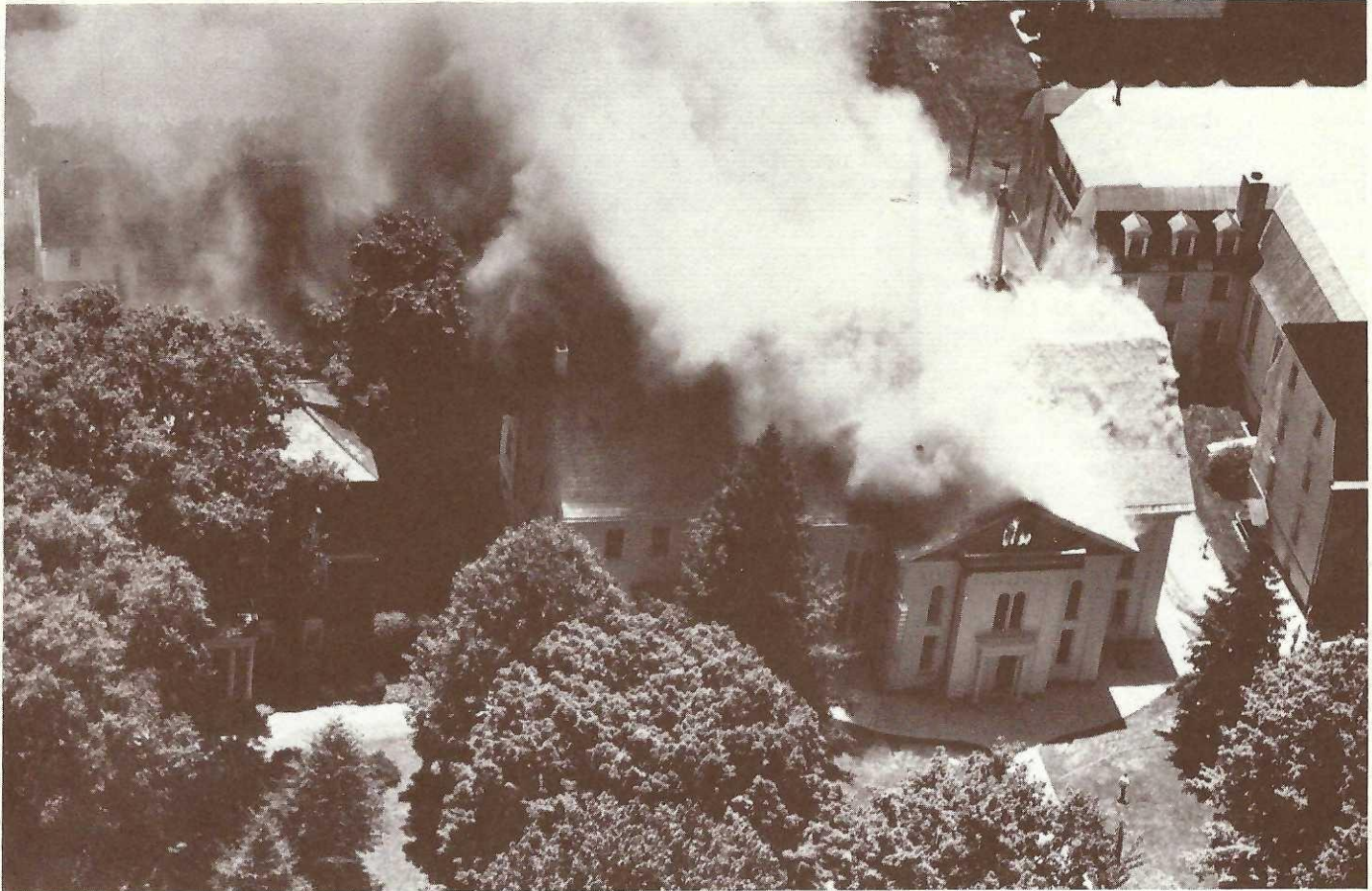
Smoke billows from the historic Lititz Moravian Church, ablaze from a painter's blow torch.
